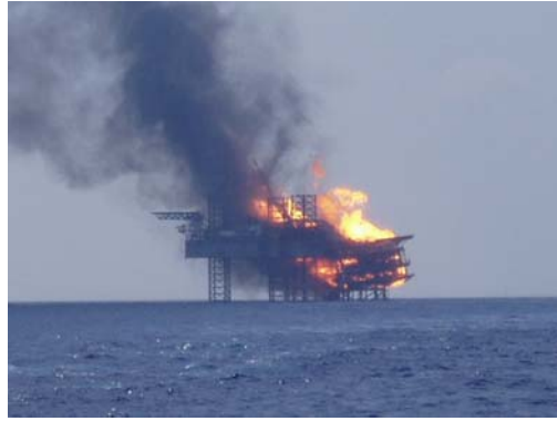
August 2004, Offshore platform accident due to a blow-out off the Egyptian coast
